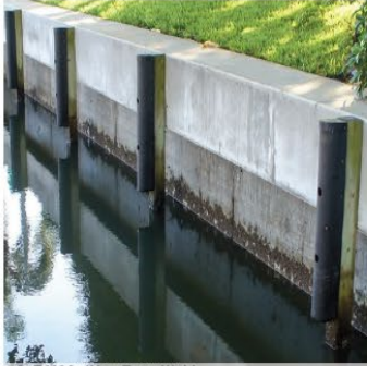
BOAT MOORING AT SEAWALL
