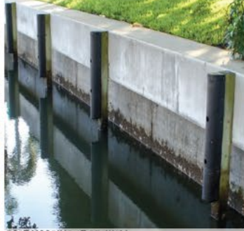
BOAT MOORING AT SEAWALL
