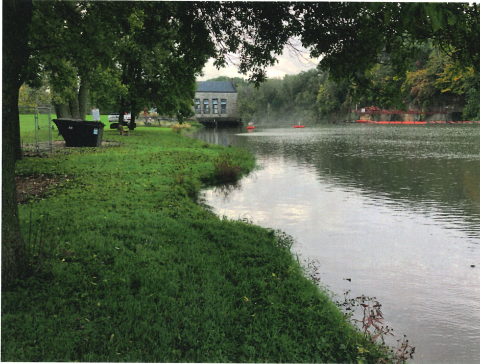
Figure 6: River Bank Erosion, View 2
