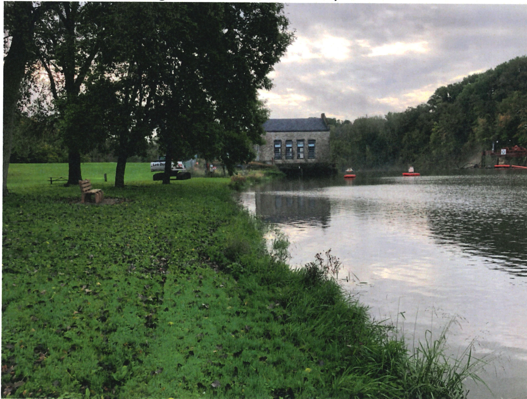
Figure 7: River Bank Erosion, View 3
